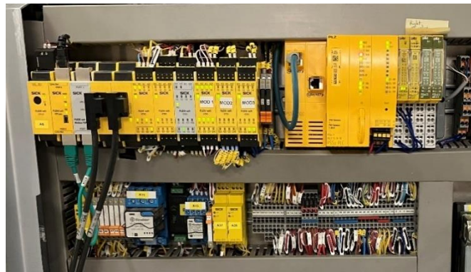
Figure 41: Safety PLC with safe IO modules
