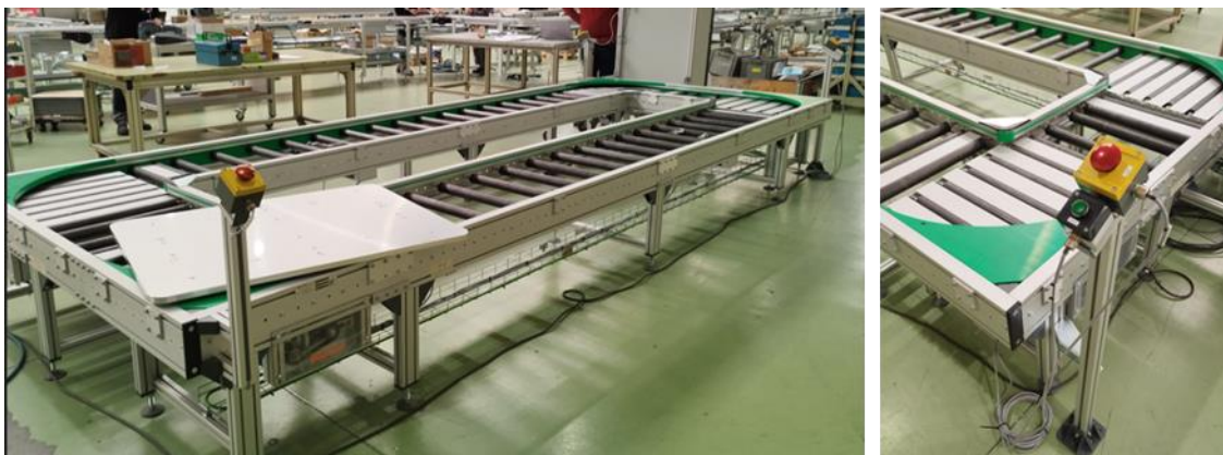
Figure 5: Conveyor's emergency buttons
